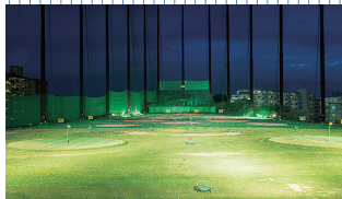
Sports Facility Lighting
